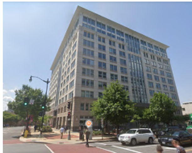
77 K ST NE IRS BUILDING
