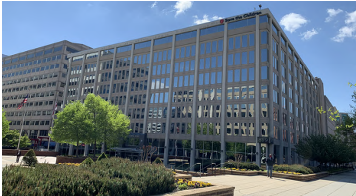
3 ACROSS NORTH CAPITOL STREET - VIEW LOOKING SOUTHWEST
